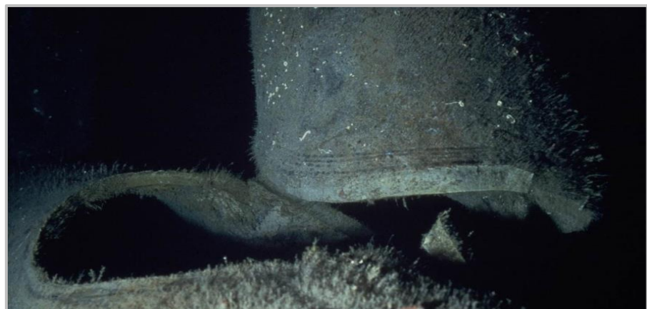
Significant Integrity Failure found by Advanced Subsea 7 ROV
