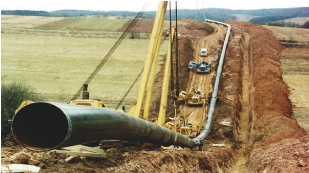
On-land metallic structures
