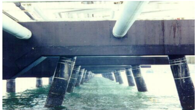
Marine metallic structures
