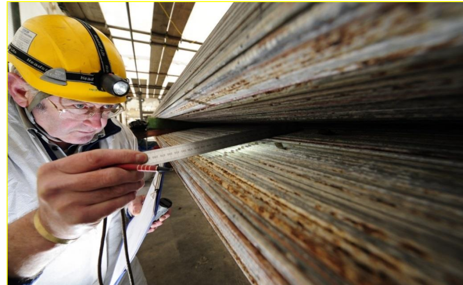
THE 'NEARLY BROKEN' BRIDGE OVER THE FORTH: Cable Corrosion
