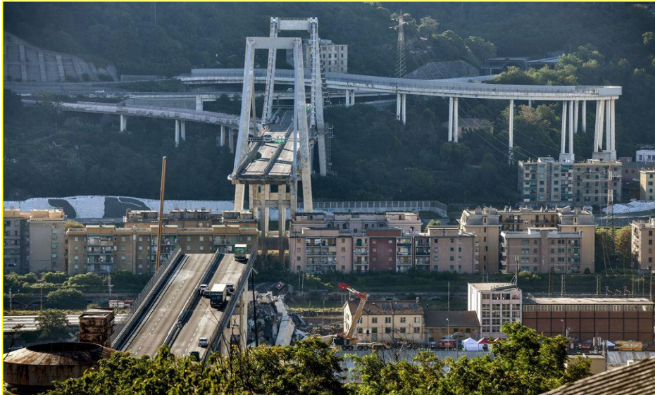
THE 'BROKEN' BRIDGE OF ITALY: Severe External Corrosion
