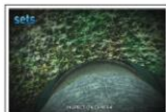
MARINE GROWTH REMOVAL & VISUAL INSPECTION OF CONDUCTOR SURFACE DOWN TO GUIDE, VIEW INTO ANNULAR GAP
