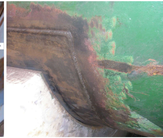
Pipe support erosion/corrosion
