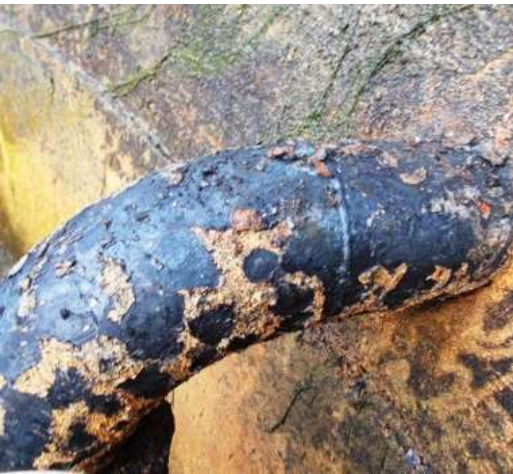
Thin-wall and pitting
