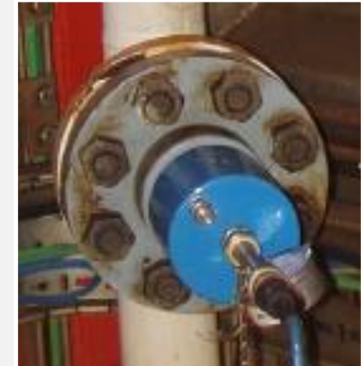
Probe Fitting with Pressure Gauge (for checking Primary Seal) and Heavy Duty Cap (for Secondary Pressure Containment)
