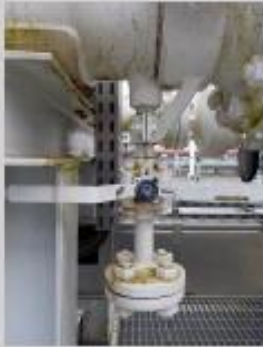
DL1 - Coating in good condition.
