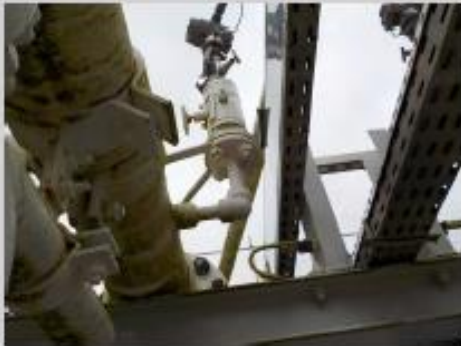
DL4 - Coating in good condition.
