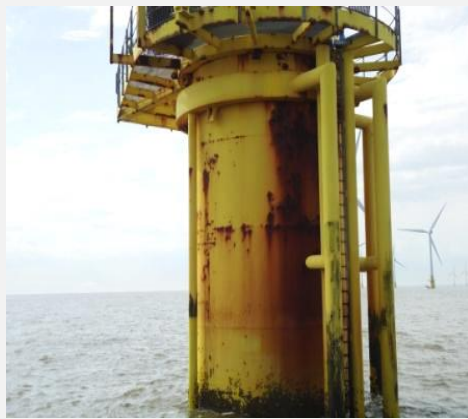
Coatings Failure
