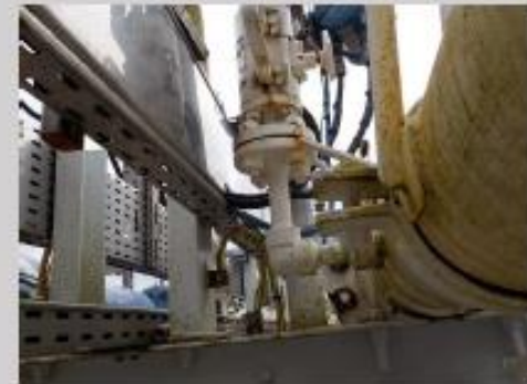
DL3 - Coating in good condition.
