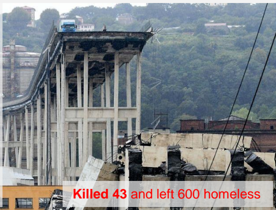
The Broken Bridge of Italy – RC Failure
