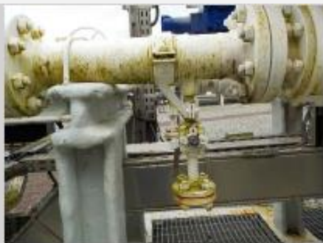
DL1 - Coating in good condition.
