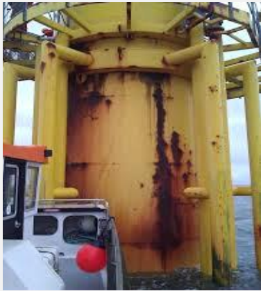
Coatings Failure
