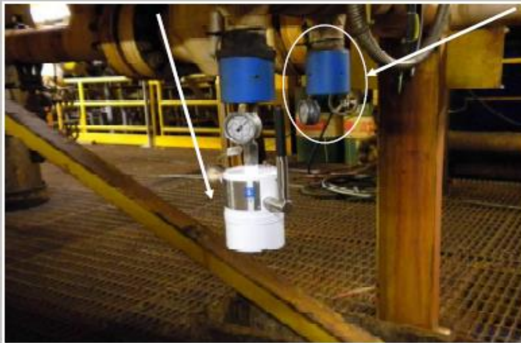
Gas Import – BOL Transmitter (White) / ER Probe and HD Cap (Blue)
