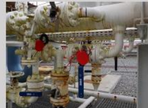
DL6 - Coating in good condition.
