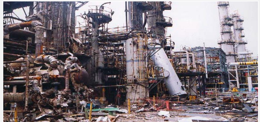
Gas Explosion – Damage Adjacent Plant
