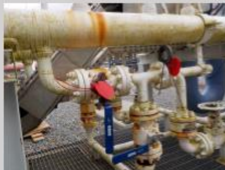
DL2 - Coating in good condition.
