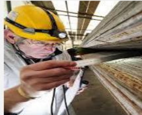
Forth Road Bridge Cable Corrosion
