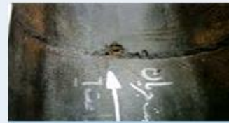
Pref.Weld Corrosion
