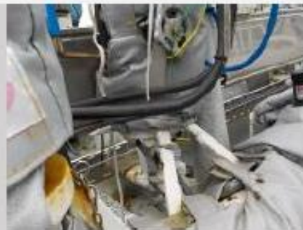
DL3 - Partially under insulated jackets.
