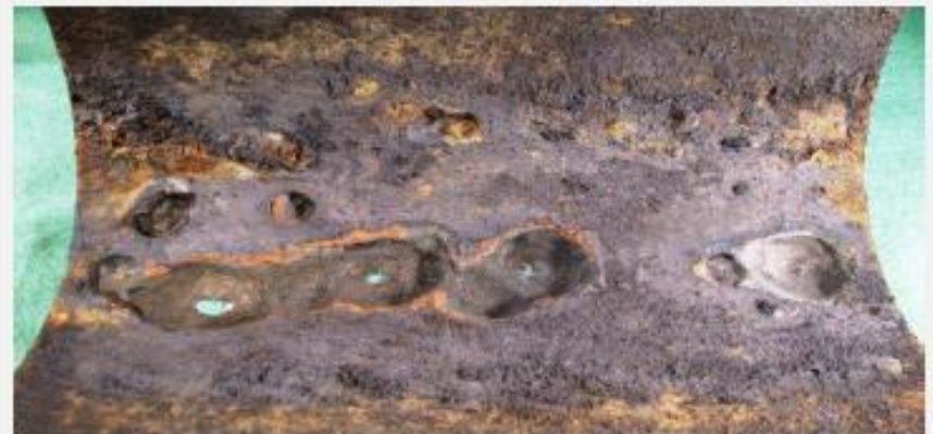
Close-Up of Pitting
