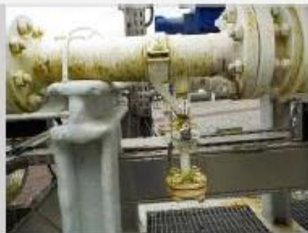
DL1 - Coating in good condition.
