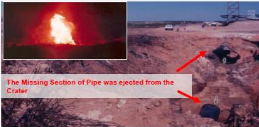
Gas Pipeline Failure – New Mexico 2000
