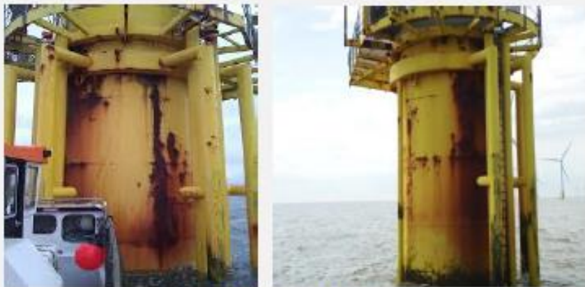
Coatings Failure
