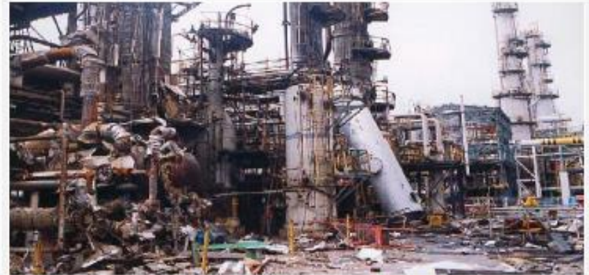
Gas Explosion – Damage Adjacent Plant
