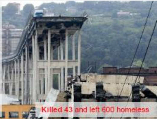
The Broken Bridge of Italy – RC Failure
