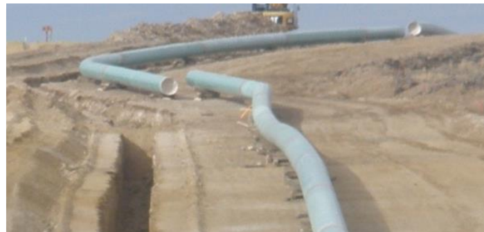
Green River, Wyoming construction site with Pipeclad 2000 & Flowliner
