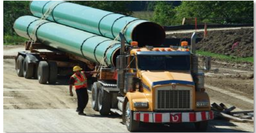
Coated pipe unloaded at Parkway
