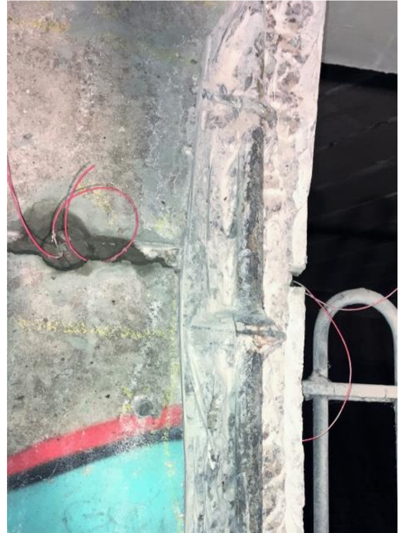
Installed Fusion™ Anode
