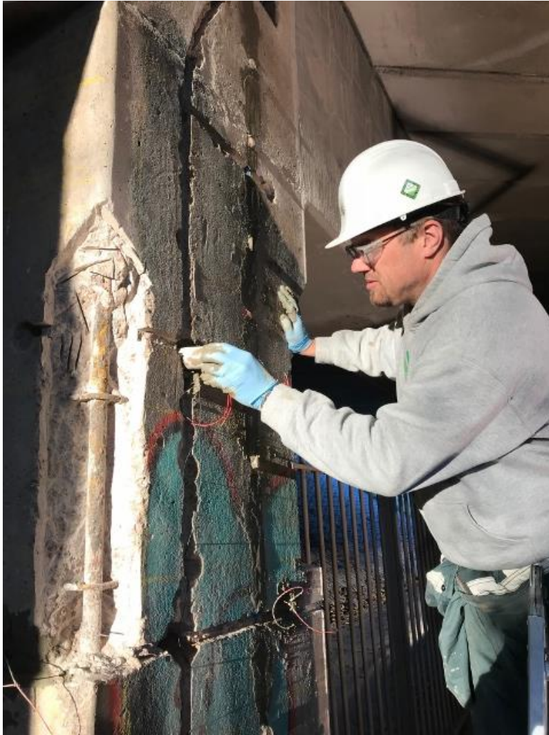
Installation of Fusion™ Anode
