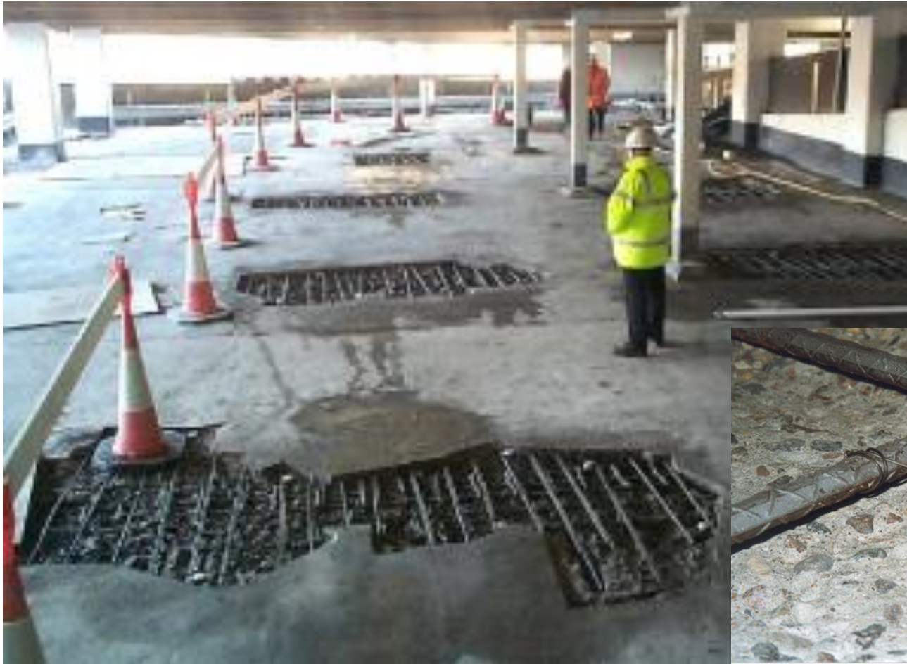
Installation of anodes
