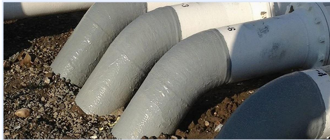
Soil to air interface pipe corrosion repair ( www.banksindustrial.com )
