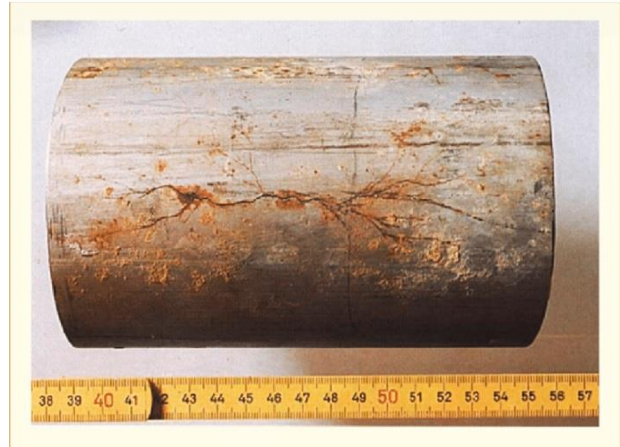
Example of stress corrosion cracking of a Type 316 stainless steel under thermal insulation at 50 to 60°C. Rinsing water containing 60 mg/lit of chloride and residual stresses are at the origin of cracking ( www.researchgate.net )
