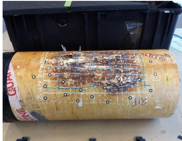
Inspections beneath corrosion scabs
