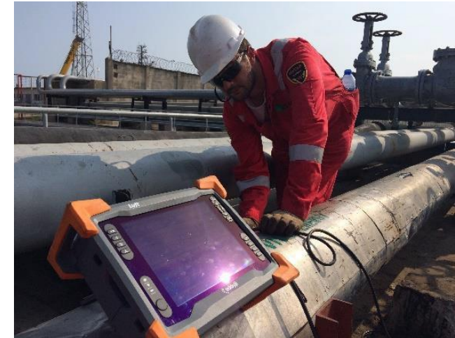
Corrosion under insulation (CUI) inspections
