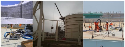
CWL GROUP Inspected 80m Crude Oil Storage Tank Floor SONOMATIC
