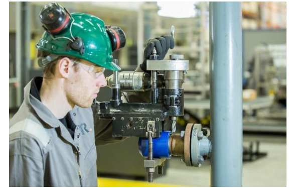
Access Fitting Refurbishment / Decommissioning Services
