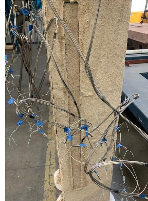
Interkote SFR@28mm LWC repair
