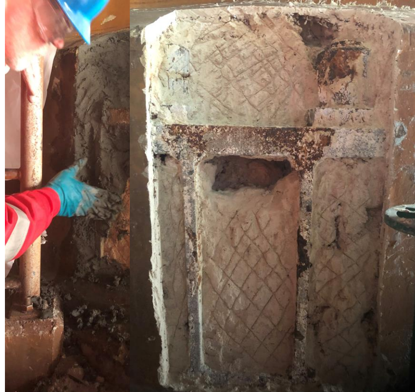
Simple hand application of Interkote SFR
