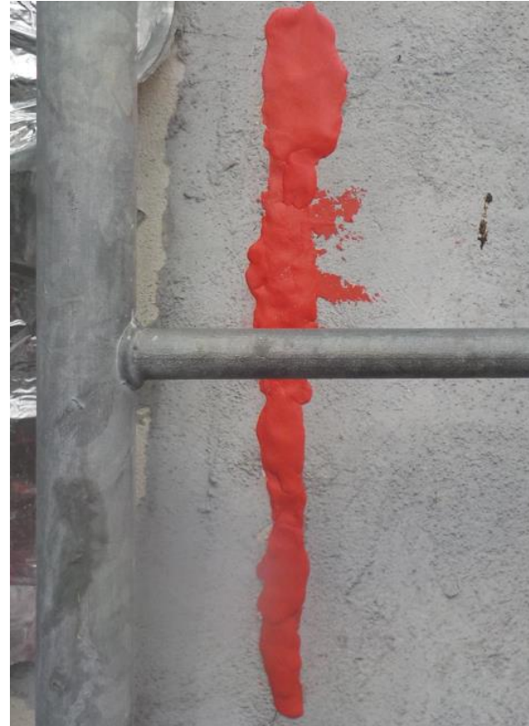
Finished IK MP repair
