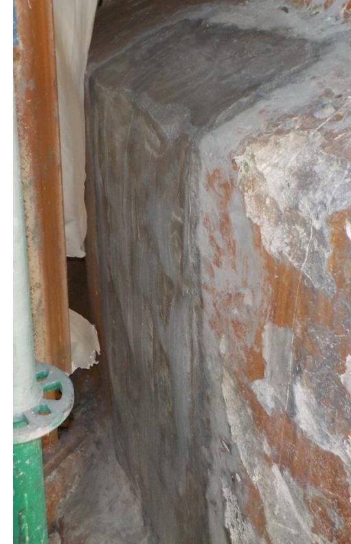
Interkote SFR finished repair
