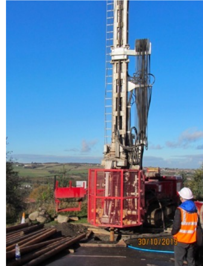
Drilling for mine water heat, Stanley Co Durham, Photo by S. McDonald
