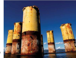
Excellent corrosion protection provided by Interszone 1000 after almost 30 years
