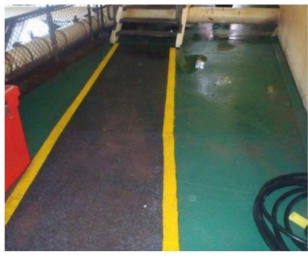
Not only providing corrosion protection this coating repair was used to level the deck to prevent water pooling which is an added hazard in winter to become a slip hazard when it freezes.
