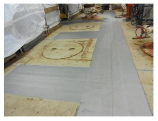
A closed circuit unit was used here to provide extremely high quality surface preparation with no dust or clean up required
