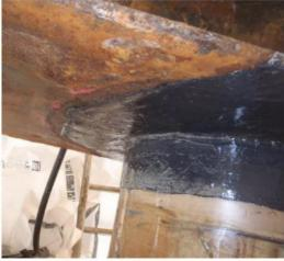
This crevice in the splash zone was of particular concern due to high pressure line with no inspection data in the crevice. Blasting was not an option as it wasn't confirmed as safe — coating system used to create profile to apply robust liquid rubber coating to protect area
