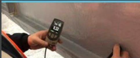
Fireproofing Coating Inspector
