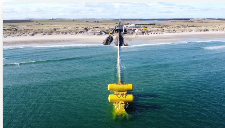
Wick Fabrication Site, UK
