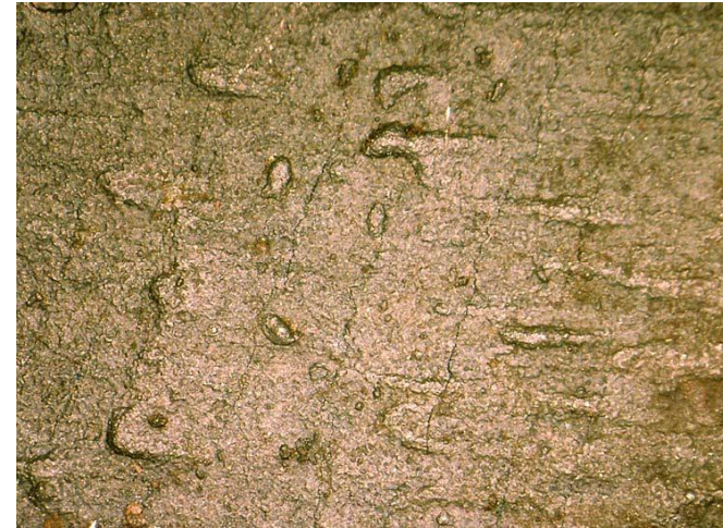
- Internal surface – mill scale - x40 mag
