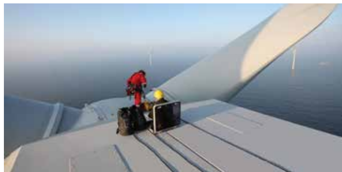
Figure 7: Wind Blade Inspection.
