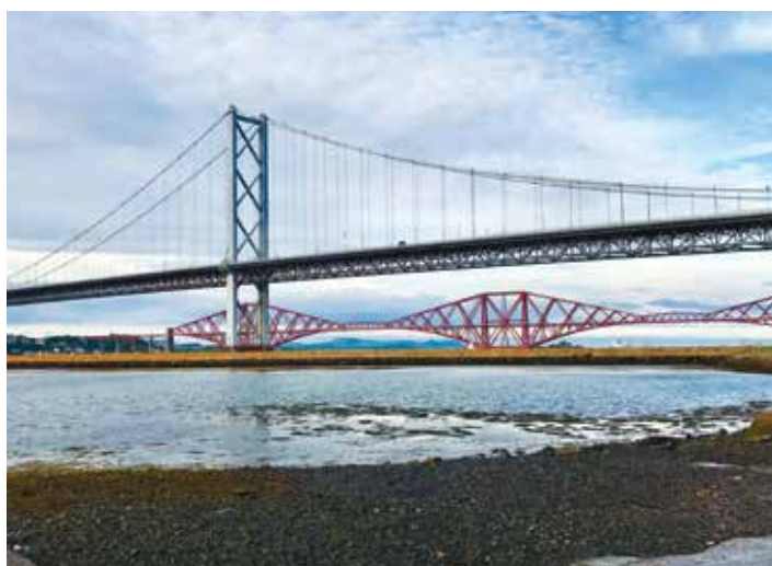
Photo 2: Forth Road Bridge, Scotland (source: Private Collection).
