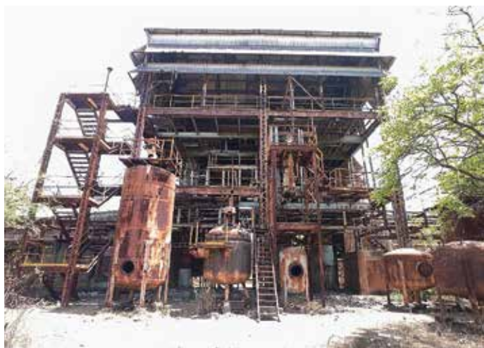
Photo: Site of the Union Carbide Disaster in Bhopal, India. It is considered by many to be the world's worst ever industrial tragedy. Corrosion was a significant contributing factor to an explosion at this insecticide plant in October 1984, which led to the release of a large cloud of toxic gas. The final death toll was estimated to be between 15,000 and 20,000.
