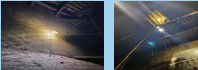
Photos: Tank Inspection - Image Courtesy of ScoutDI.
