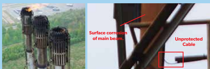
Photos: Flare Stack Inspection - Image Courtesy of Vysus Group.
