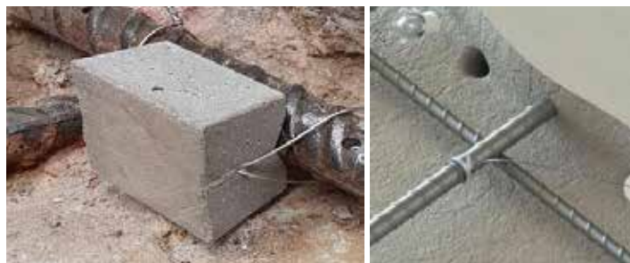
Photo: Precast Anode (Left) Attached To The Steel Within A Patch Repair During Installation And Discrete PatchGuard™ Anode Schematic (Right) Showing Its Installation Into The Periphery Of The Patch.
