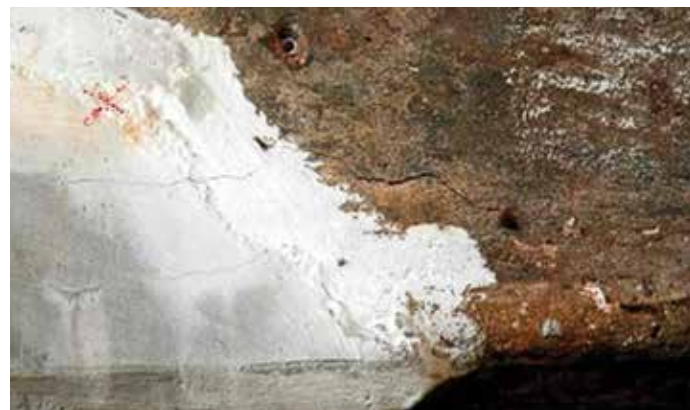
Photo: Patch Repair Cited as Being Protected By Precast Galvanic Anodes in 2015.
