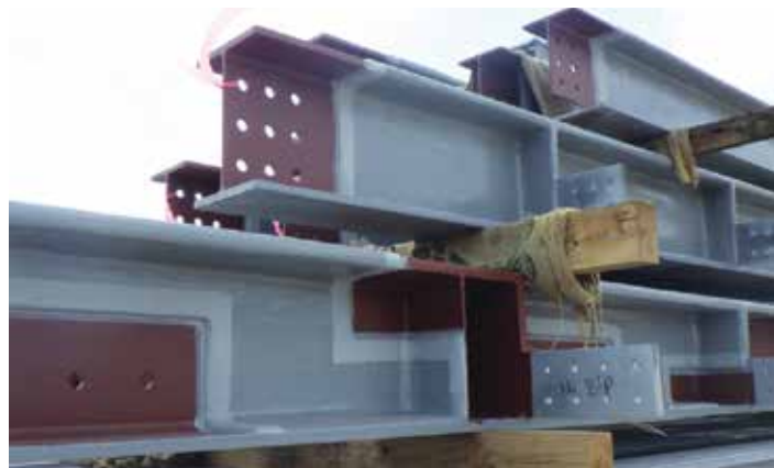
Photo 1: An Example of Galvanised Steel Section with EPFP Applied Ready for Transport.
