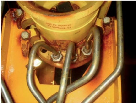
Figure 9: Umbilical connection showing severe corrosion(source: EEMUA Publication 194)
