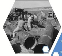
1960s - Saw the birth of mainline coating systems. FBE also provided excellent flexibility properties, this was an answer to the <u>failures</u> of many previous materials due to handling and bending of the pipe spools during pipelay and subsequent cracking of the system
