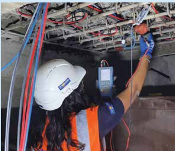
Photo: Cathodic Protection in Concrete Monitoring.
