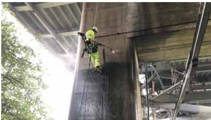
Photo: RAT Based Pressure Cleaning Activities.
