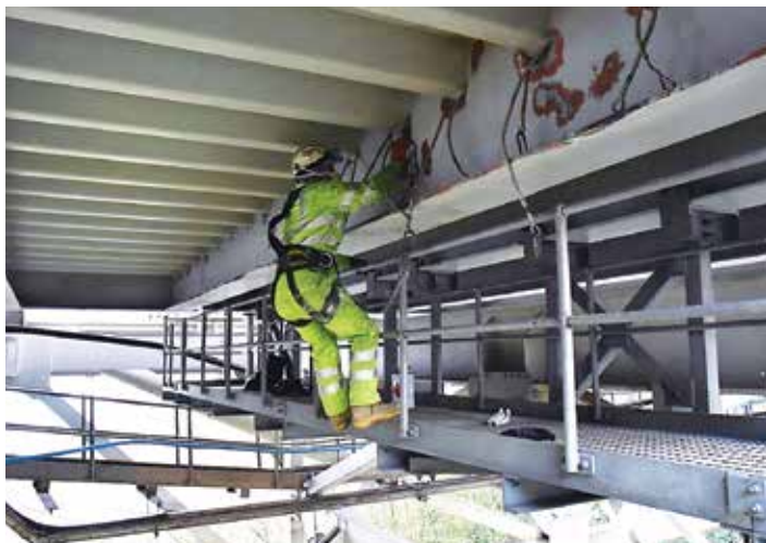
Photo: Distance Harness Assisted Solvent Wash Under Deck.
