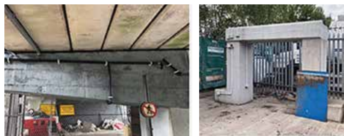
Photo: Slide Concrete Conductive Anode Paint Trials.
