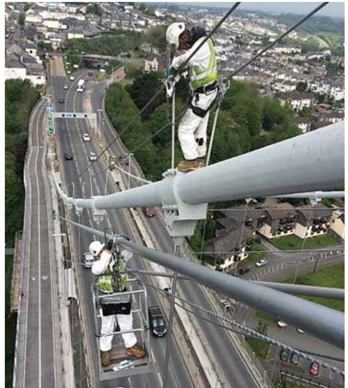
Photo: Incline Cable Painting.
