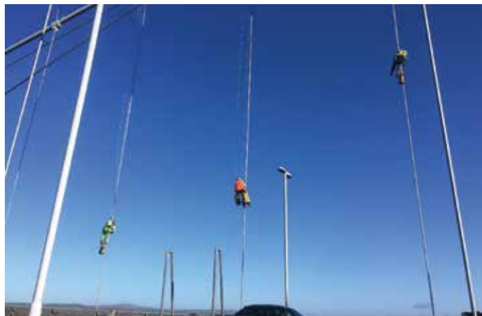
Photo: Bridge Hangar Painting.
