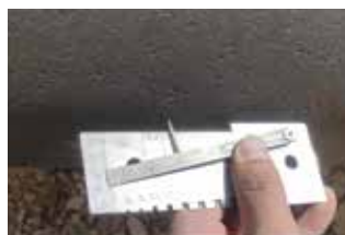
Figure 7 (b): Direct Examination Photos [1].
