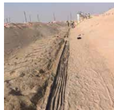
Figure 5: Installation of CP Cables in The Same Trench of the MMO Linear Anode.
