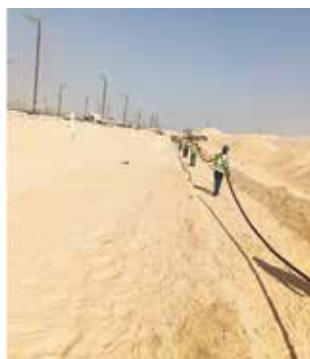
Figure 4: Installation of the MMO Linear Anode.
