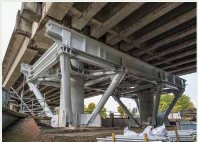
Photo: One of 23x Temporary Props Required for Repairs to M8 Woodside Viaduct, Image Courtesy of ALAMY.
