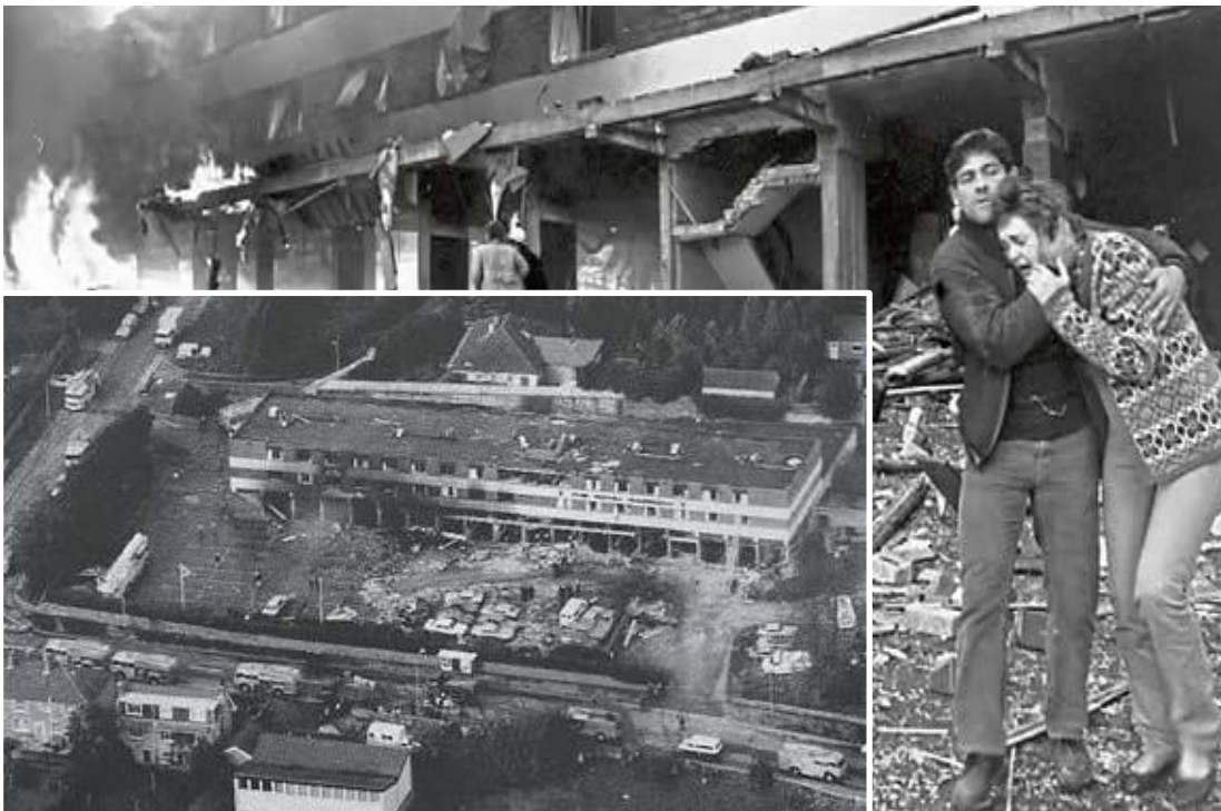
Explosion severely damaged the Hotel which was later demolished.
