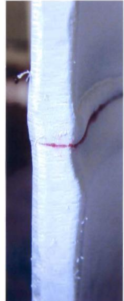
Figure 4: Crack revealed by DP-across thickness.
