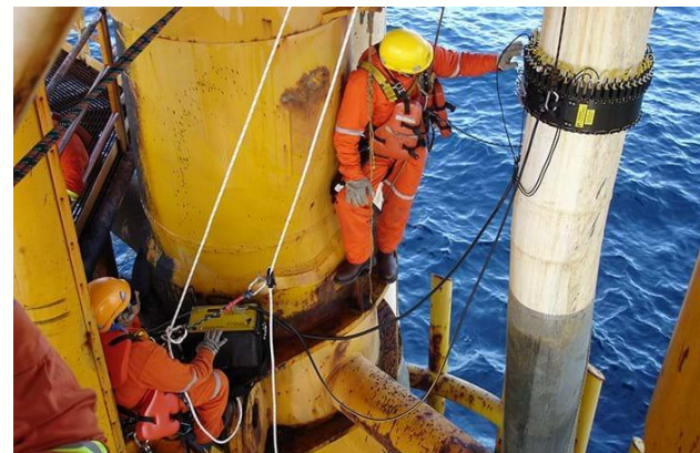
Offshore inspection via rope access
