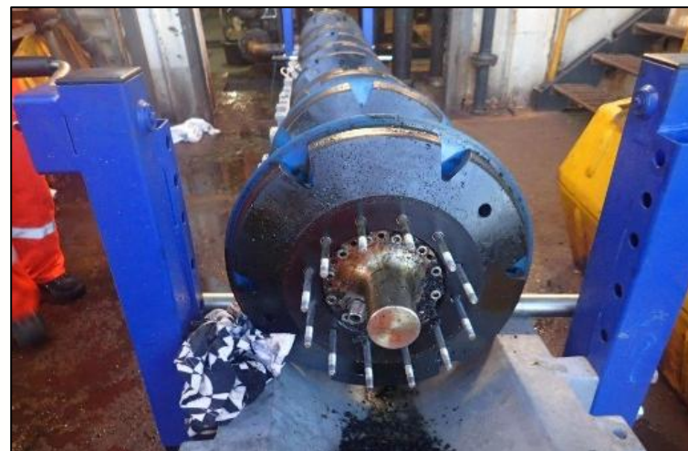
Inline pipeline inspection using NDT
