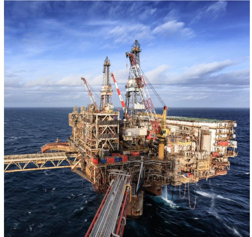
Aging offshore oil and gas platform
