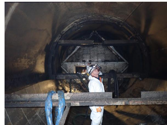
Internal of a pressure vessel
