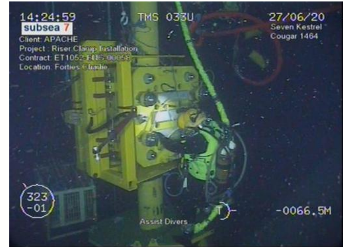
Subsea clamp installation
