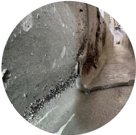
On-Site Survey, Condition / Integrity Assessment
