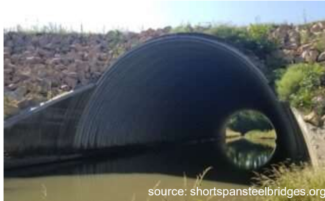
Buried Steel Bridge
